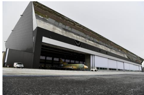
Mérignac – Multifunctional production facility
