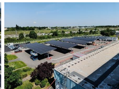
Poitiers – photovoltaic panels
